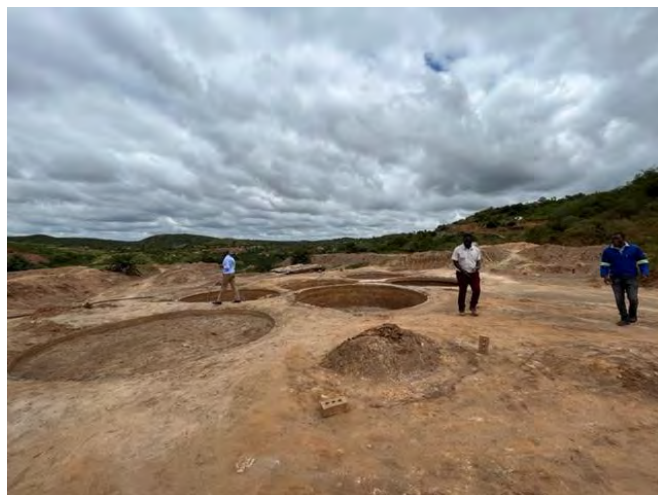
Photo 7 : Leach tanks on the tailings.
