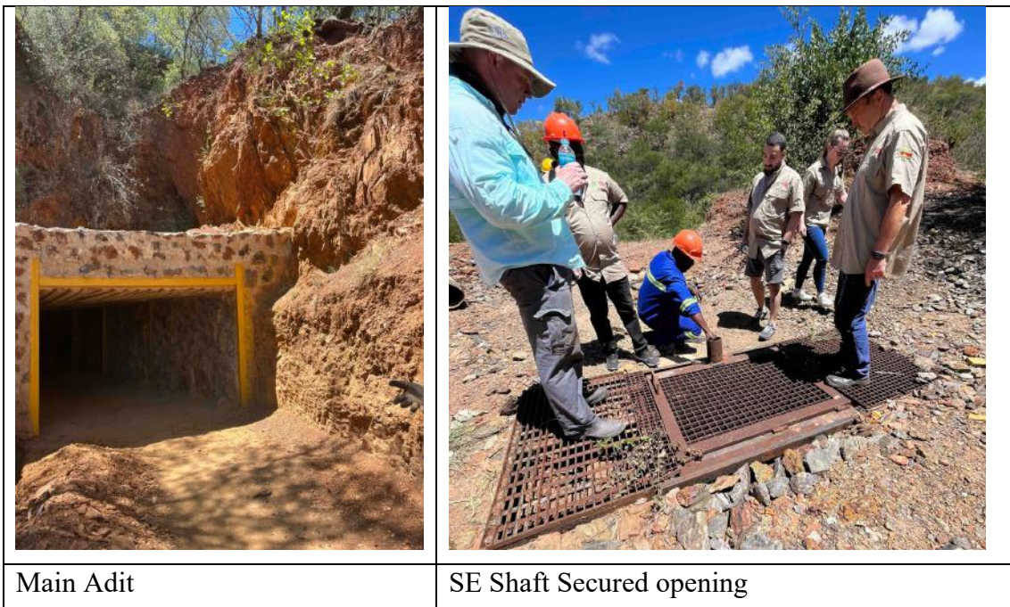
Photo 7: The Surface Expression of the 2 Mining Shafts on site.
